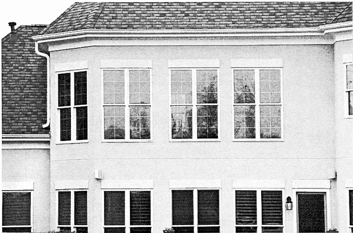
This “single eyebrow” is a common practice with stucco homes, and will no longer be approved by the ACC.
